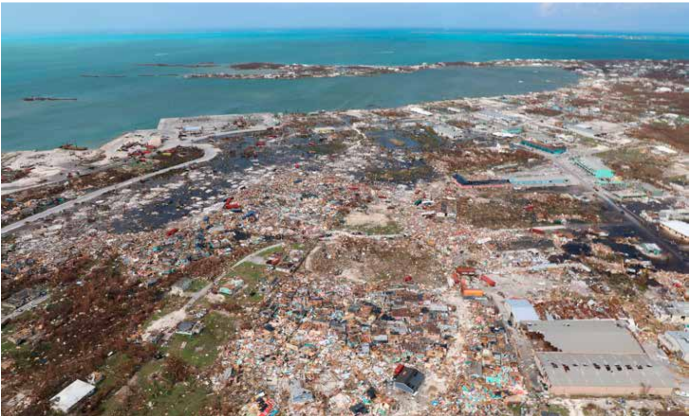
Widespread destruction caused by Hurricane Dorian is seen from the air, above Marsh Harbour, Great Abaco island, on September 4, 2019. (Gonzalo Gaudenzi/AP)
